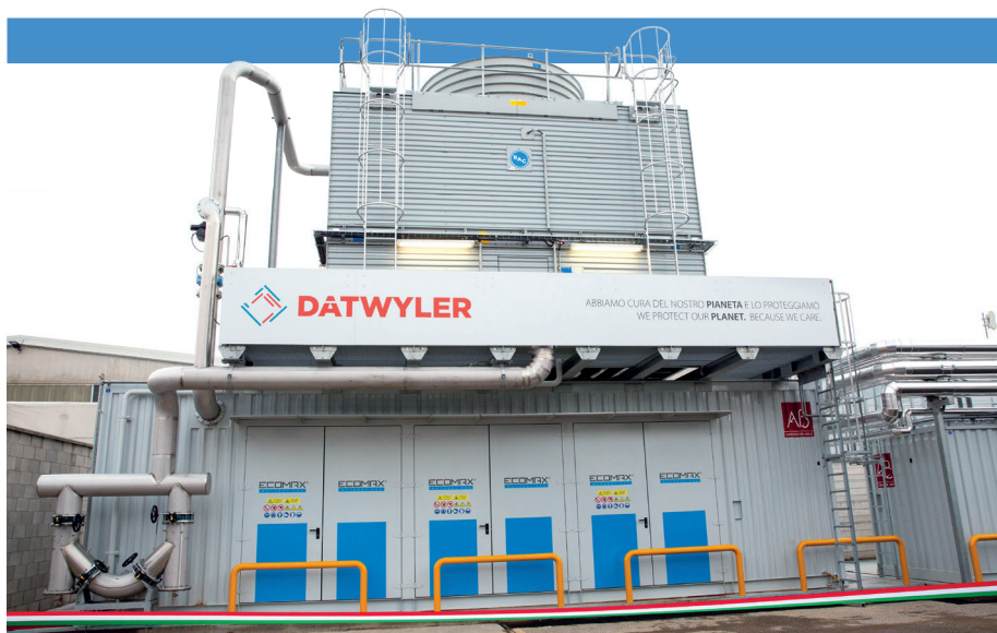
Figure 1: A modern trigeneration unit at Datwyler's plant in Italy reduces the company's CO 2 emissions by 900 tonnes per year.
